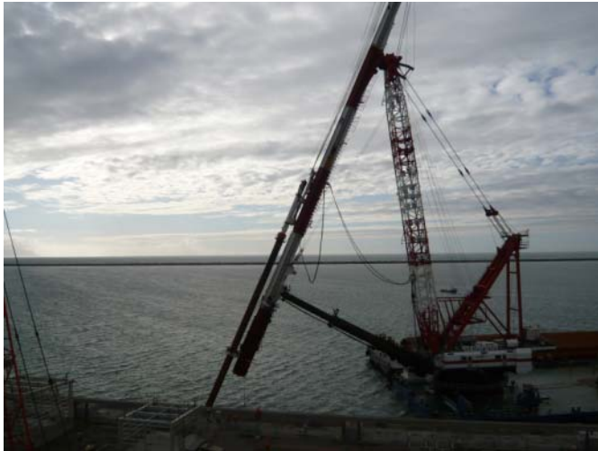
Piles with angle
