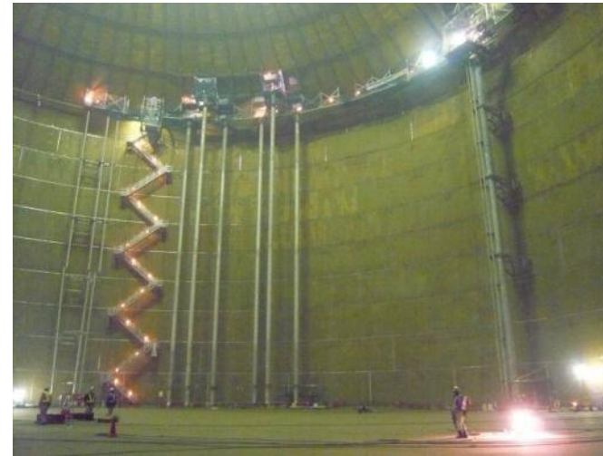
Inside of tank
