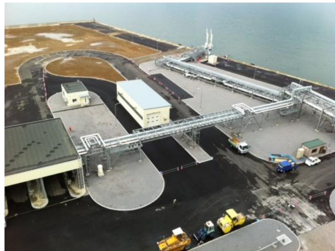
Coastal shipping berth & truck scale for lorry
