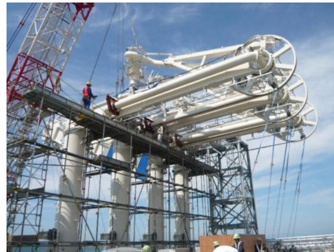
Installation of arms
