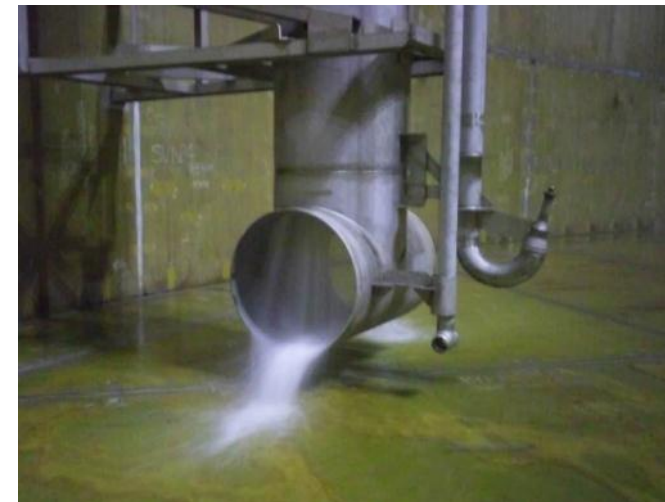
Starting to water injection for loading test
